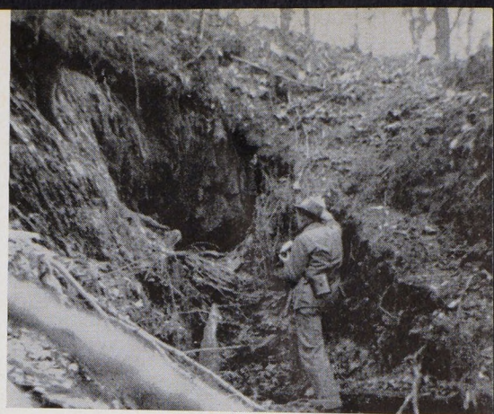
A modern prospector inspects the horizontal shaft entrance to the Rooks Mine, for many years now blocked by fallen rocks.
